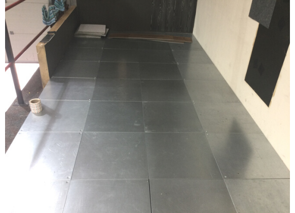
Raised metal access flooring after uplifting flooring installed using IOBAC Adhesive-Free MagTabs®
