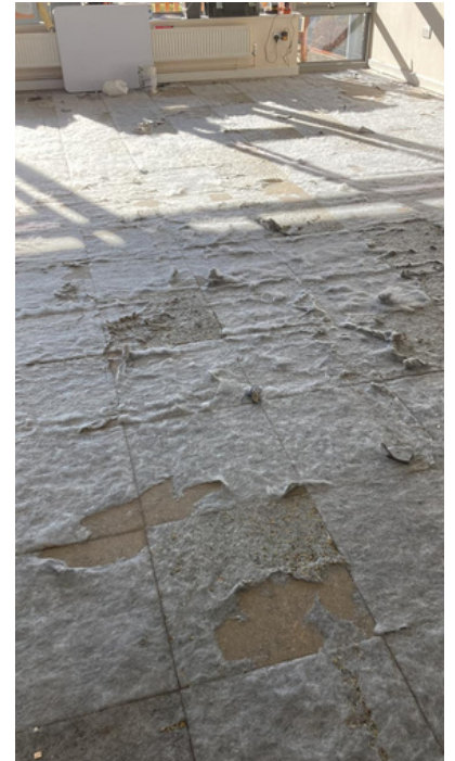
Remains of old floor covering backing stuck to sub-floor
